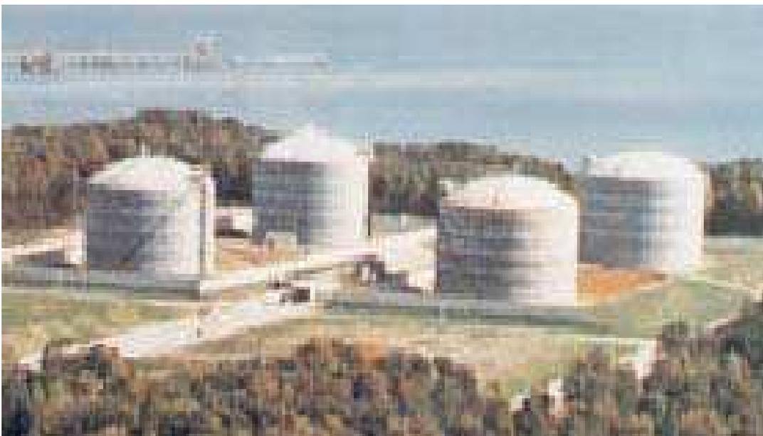
**Figure 14. Single Containment Tanks**
