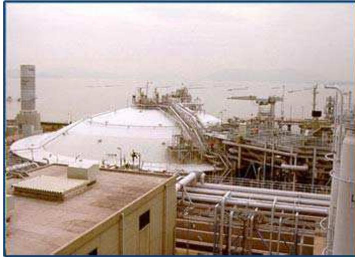
**Figure 24. In pit LNG storage tank**
